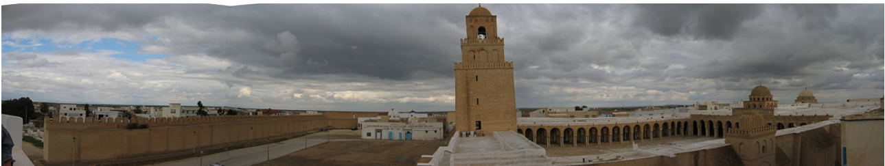
Panorama of the minaret and the courtyard (on the right)
